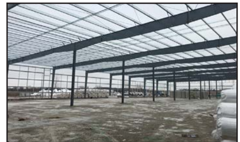
Windsor location expansion progress
